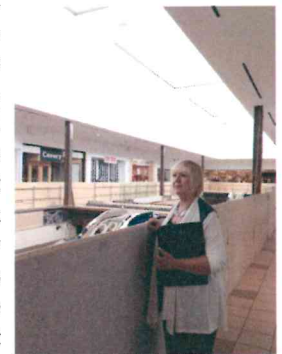
Vice President Nance MacDonald monitors renovations, EMTC
